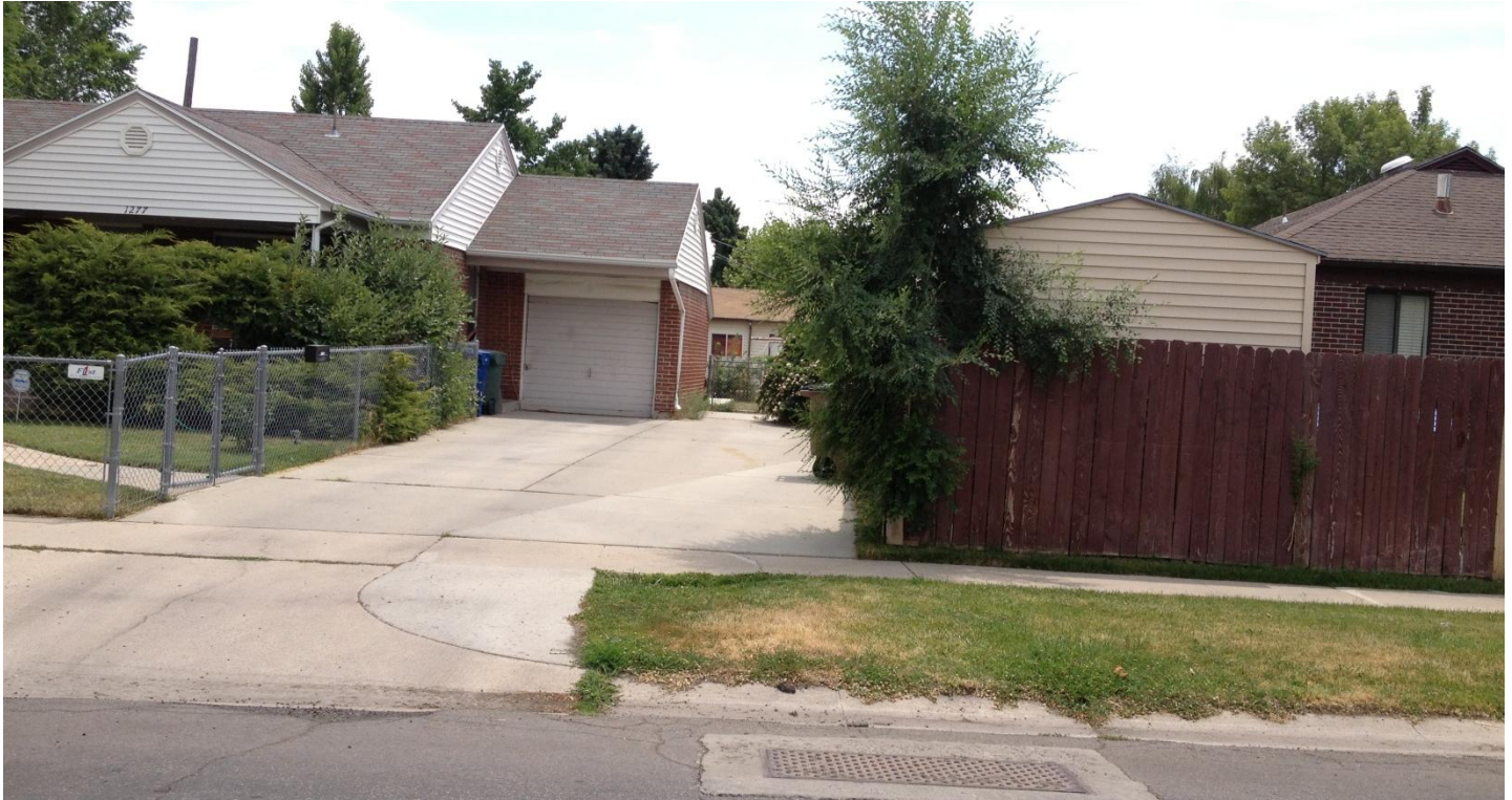
6' Corner Side Yard Fence at 836 N 1300 West. Fence is setback from the adjacent property owner's driveway by approximately 7 feet, though original driveway appears to have met 10 foot sight distance requirement. Fence extends to a point behind the front façade of the home.
