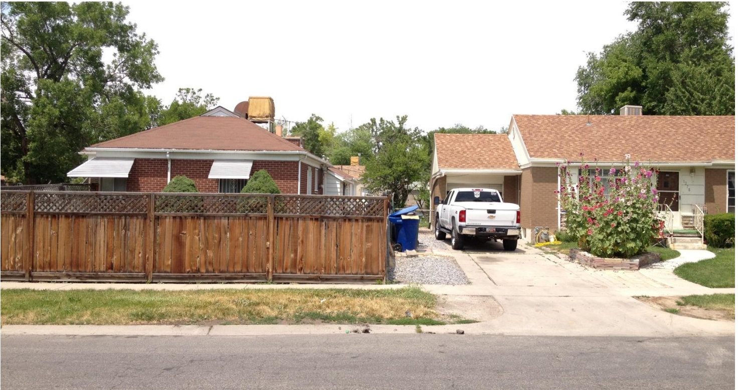
6' Corner Side Yard Fence at 858 N 1300 West. Driveway entrance is located approximately 6 feet from the fence. 6 foot fence extends to a point in-line with front façade of home.
