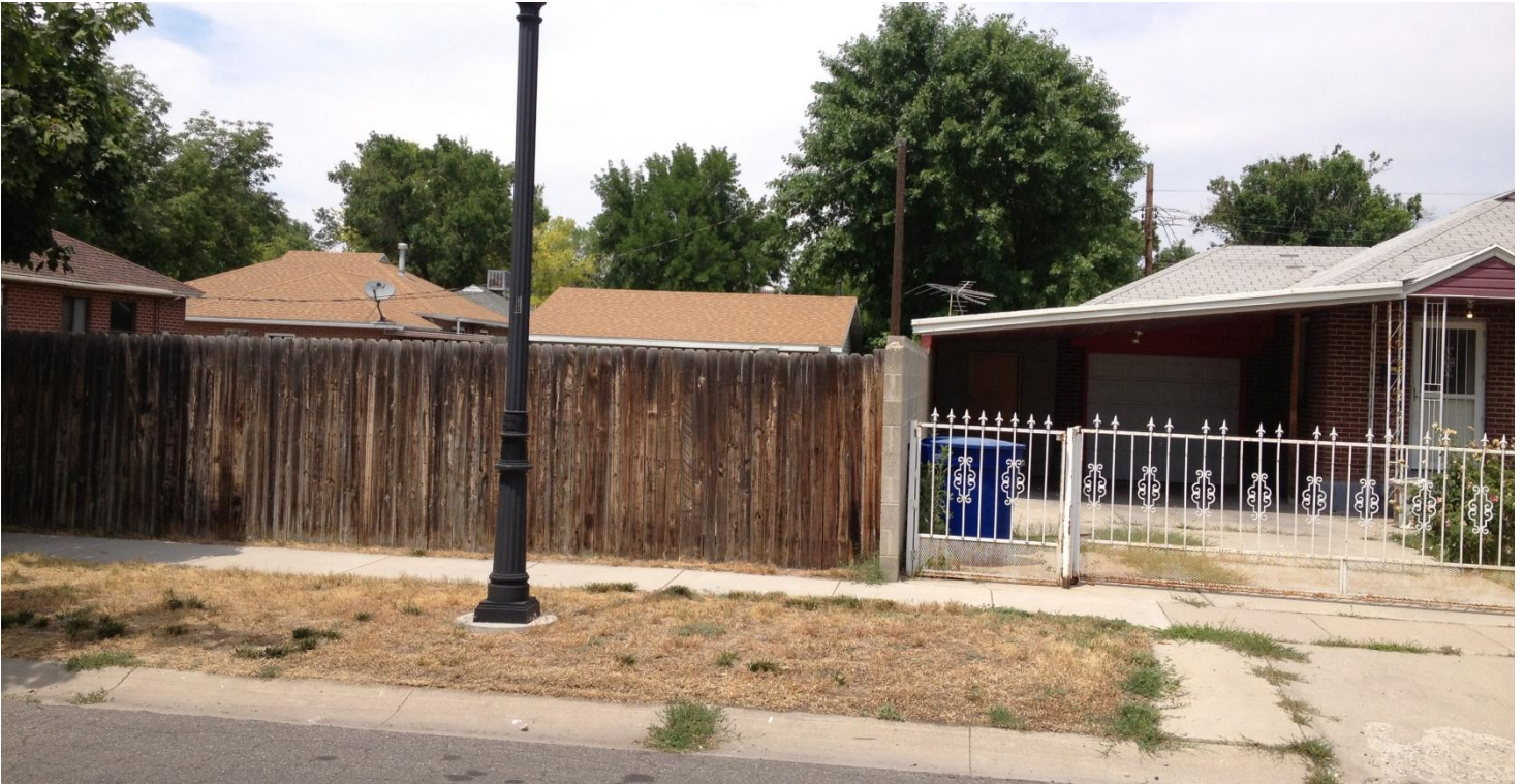
6' Corner Side Yard fence at 872 N 1200 West (on left.) The fence is setback approximately 5' from the driveway. Original driveway appears to have been 8' from fence. Fence extends to a point in-line with front façade of the home.
